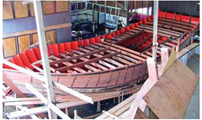
ABOVE: A fishing boat hull under construction LEFT: A traditional river boat takes shape
