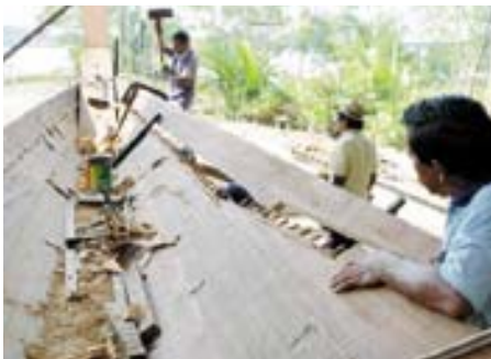
Joining two planks
