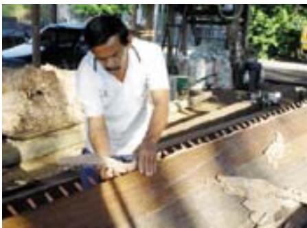
Applying the caulking bark
